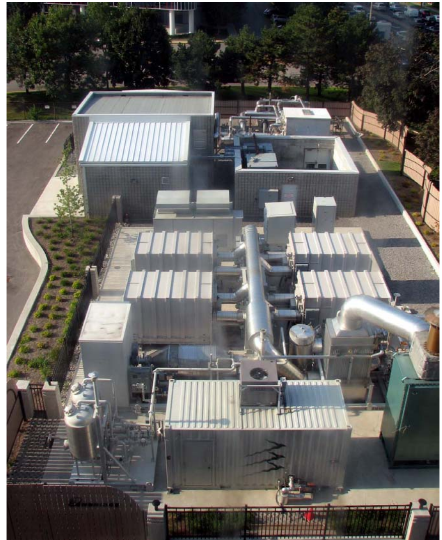
Image: Enbridge 2.2 MW Hybrid FuelCell demonstration of cleanest, most efficient gas power plant, Toronto, Ont.
